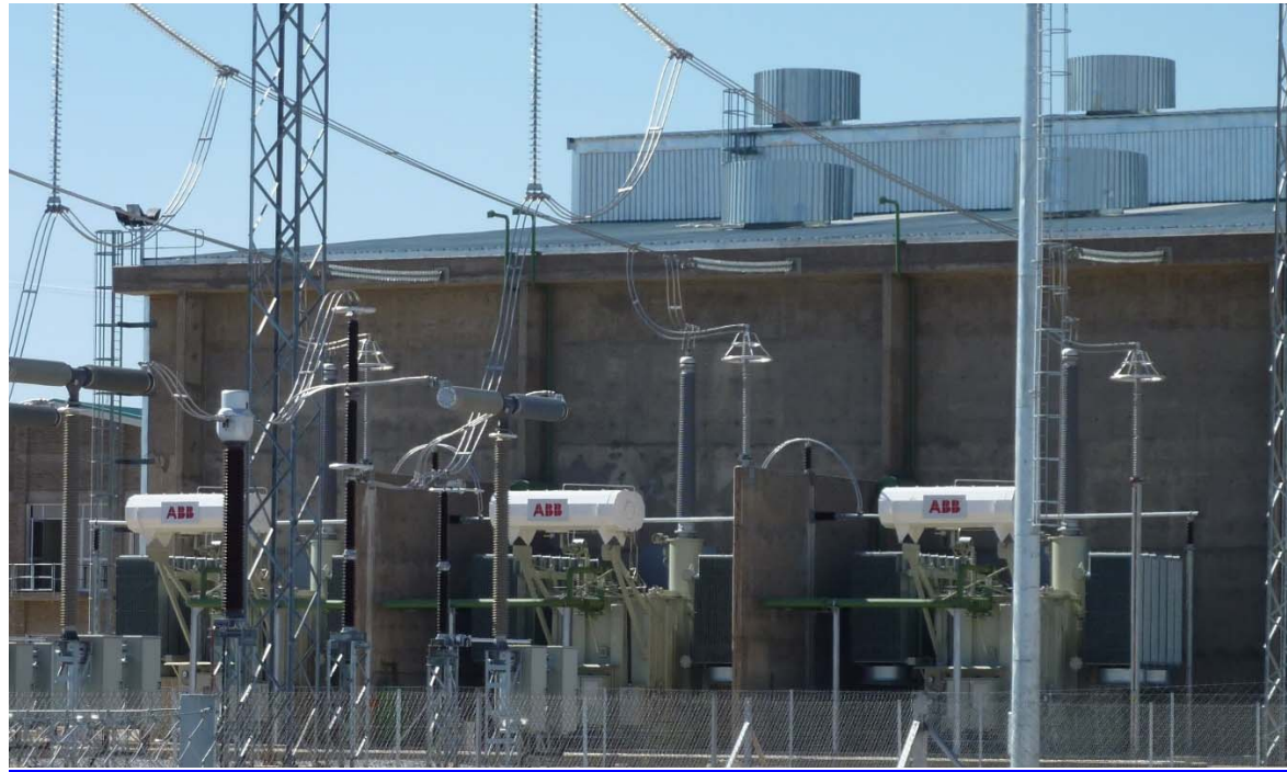
Plate 5.14 – Typical Interface transformers Image: ©ABB
