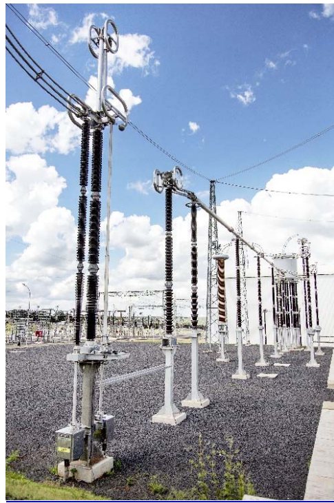
Plate 5.10 – Typical HVAC Disconnector Image: ©ABB
