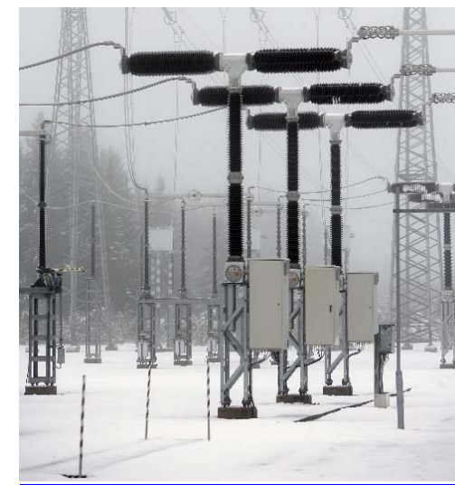
Plate 5.9 – Typical HVAC Circuit Breaker Image: ©ABB
